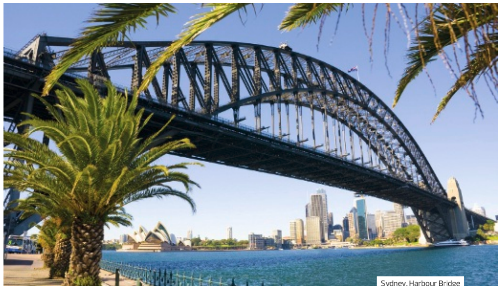
Sydney, Harbour Bridge
